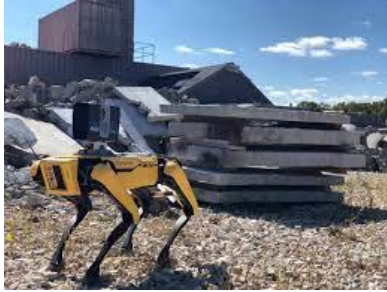
fig(i) robots in construction site
